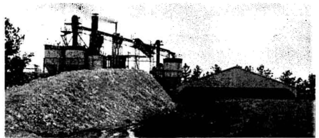
Stockpiles of East Texas bentonite (left) and filter clay (right) are draglined into building (rear), run through grinder, then fed into drier.
