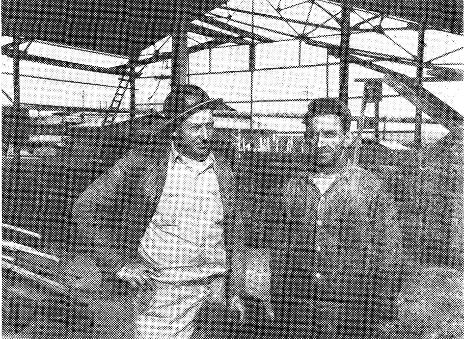
GARVIE WALKER AND WELDON BOWMAN are caught at the end of the dry sorter while the building was under construction. Walker is construction foreman and Weldon is a mechanic in the truck shop.
