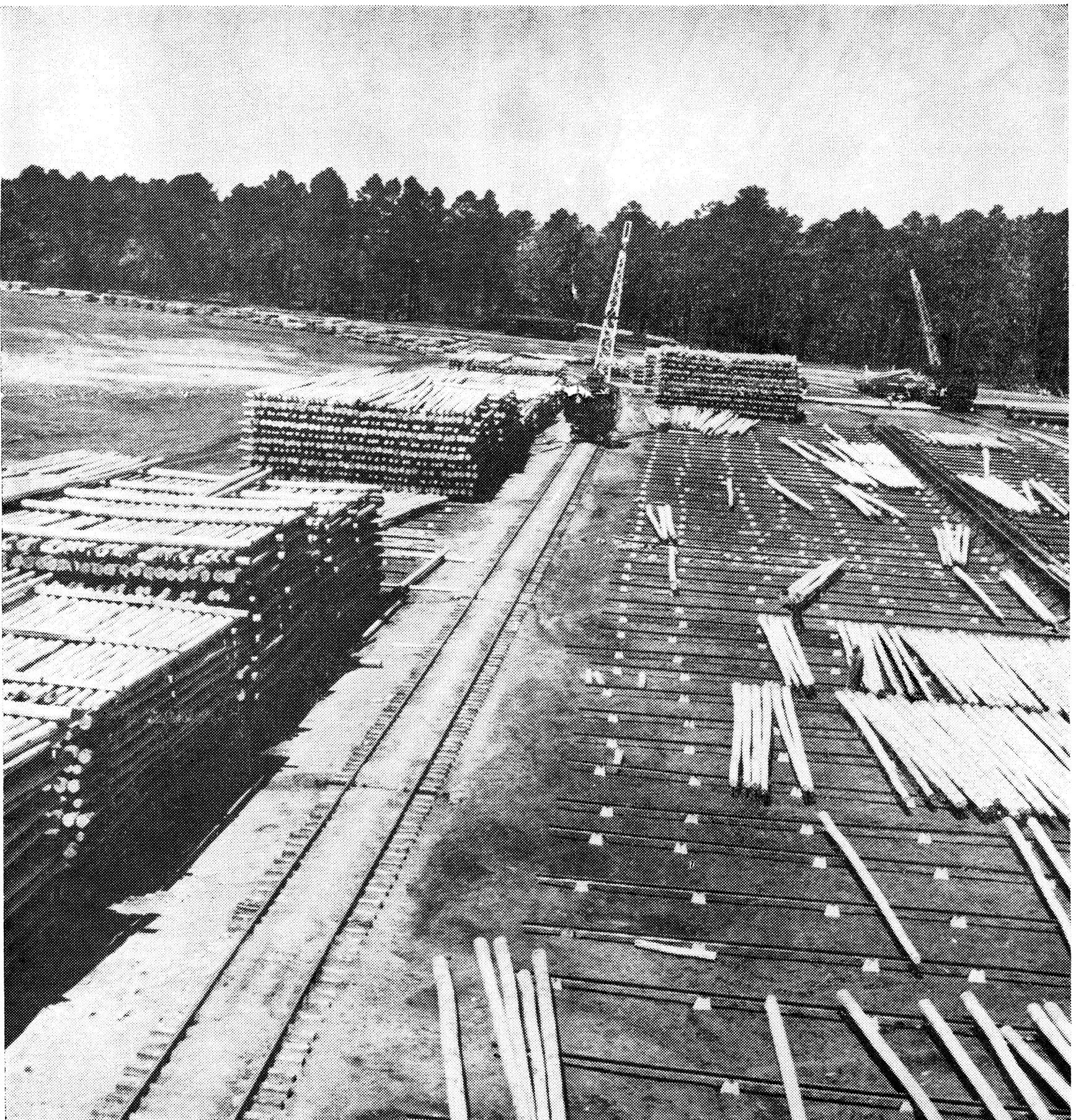
THE WESTERN END OF THE POLE YARD gleams brightly as one of the most well developed yards in Treating Division circles. This one of the Southern Pine's Treating Division Yard ranks as tops with its two new cranes, 600 foot conveyor chain (extreme right), graduation skids (middle right), air drying stacks (left middle), and large supply of fence posts and ties in the extreme background.
