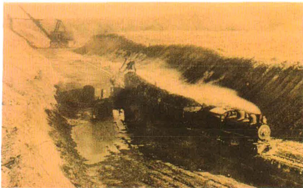
The Malakoff dragline, in the background, had a bucket capacity of eight cubic yards and was considered huge at the time. Today, draglines up to 100 cubic yards in capacity are being used by the TU System.
