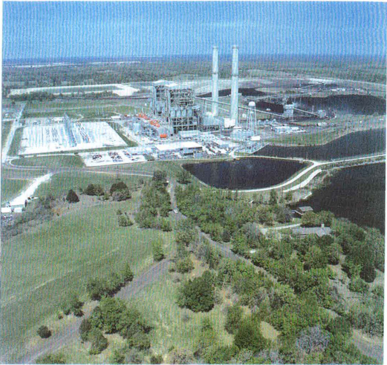
Big Brown in Freestone County, with its two 575,000-kilowatt generating units, was the TU System's first modern lignite-fueled power plant. It, like the System's other two lignite plants, includes a cooling lake and adjacent parkland. At the three locations, the System has made more than 9,000 acres of lake surface and almost 1,900 acres of land available to the public for recreational purposes.
