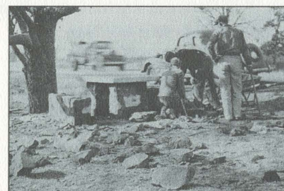
A National Youth Administration (NYA) crew builds a picnic table and bench near Gainesville.
