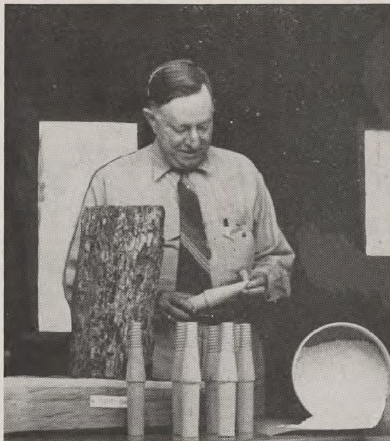
Hartwell Jalonick who helped initiate the wood research at the Texas Forest Service Laboratory, Lufkin, Texas, examines one of the treated insulator pins, made of red oak, which are now equal to bois d'arc and locust in quality.
