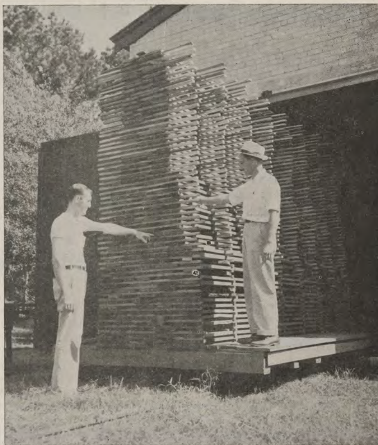
A TEST RUN of redgum lumber is shown piled in front of the dry kiln at the forest products laboratory of the Texas Forest Service where it has been dried under carefully controlled conditions. The lumber was previously dipped in a chemical solution. It was furnished by the Southern Pine Lumber Company as part of a project attempting to find ways of drying lumber faster without serious defect for war use.
