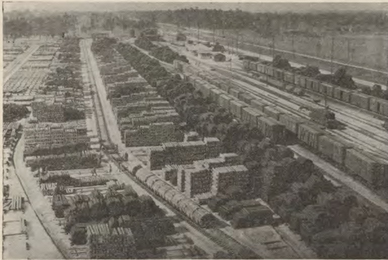
In the yard of this Texas creosoting plant, ties and poles are given preservative treatment. Fifteen plants like this one treat some 300,000,000 board feet of wood each year, furnishing employment to 2,500 workers. (Photo courtesy Texas Creosoting Company).
