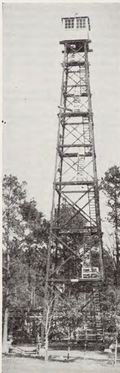
Above is a picture of the lookout tower recently completed at the Division of Forest Protection headquarters at Lufkin, Texas. The tower is built of pressure-treated creosoted timbers. The weight of the creosoted material in the tower amounts to 24,300 pounds, and the wooden material in the cab, stairs and platform landings amounts to about 1,200 pounds. The hardware, bolts, and nuts weigh an additional 987 pounds, making the total weight of the tower resting on the concrete piers, 26,487 pounds or slightly over 13 tons. The tower is 100 feet tall.
