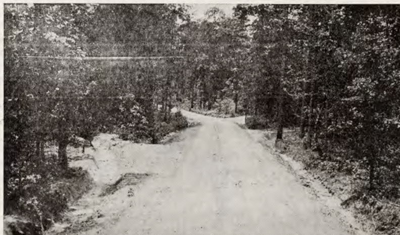
Over 2,000 miles of forest roads similar to the above have been constructed in the timbered portion of East Texas by the C.C.C. forestry camps operating under the supervision of the Texas Forest Service.
