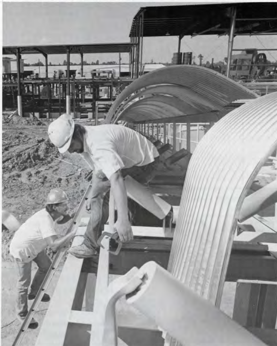
Workers assemble a bark conveyor for the Temple-Eastex sawmill project in Buna. This conveyor, completely supplied by Structural Fabrication, will run approximately 200 feet in length.
