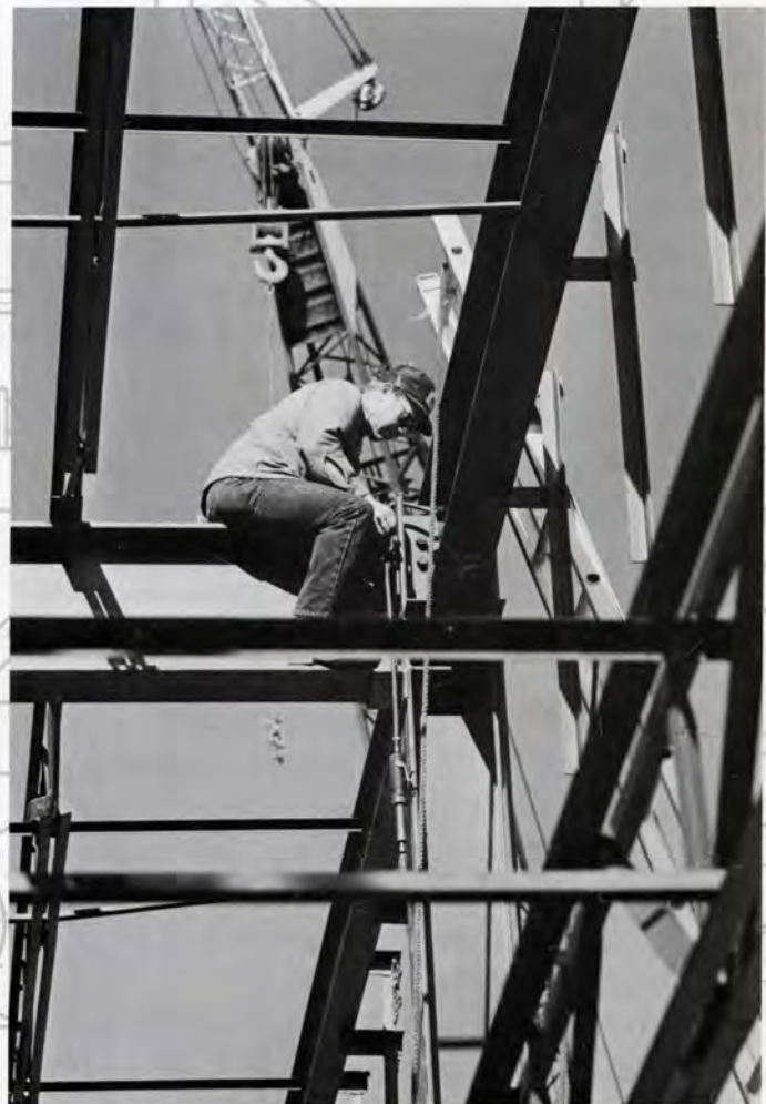
Tommy Reynolds , of the Structural Fabrication Department, aligns and tightens the bolts on the frame of One Research Plaza. The building is located at College Station, Texas.
