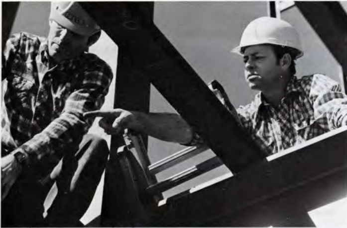
Dale Frels and Perry McKnight discuss the alignment of beams and columns which support One Research Plaza.
