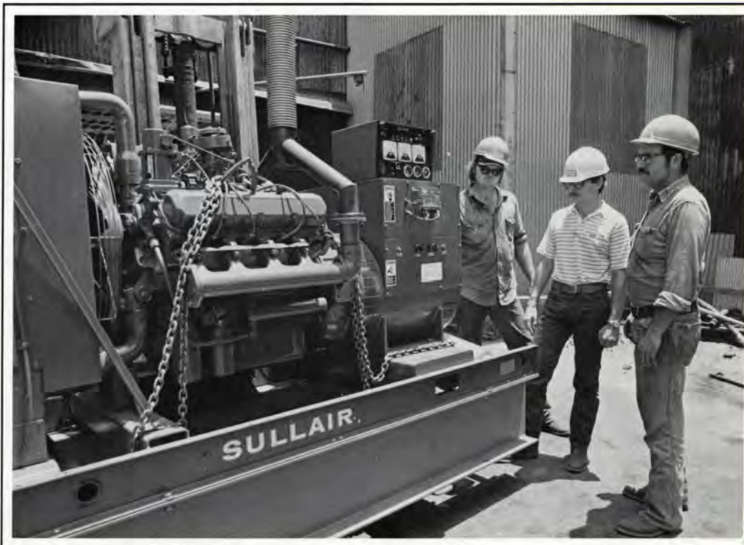
Foundry engineering employee, Jeff Lankford, center, visits with Tommy Sides, left, and Jack Russell, foundry maintenance employees, who installed the new $14,000 stand-by generator.
