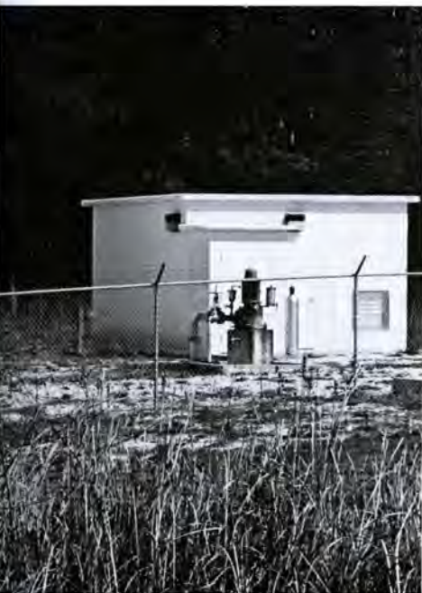
(Far left) The machine shop has established a central storage building for the bulk storage of all lubrication oils, cutting oils, greases and cleaning solvents. Instead of storing the materials in 55-gallon drums throughout the plant, necessary materials are delivered to the area where they are needed. Pictured is Joe Hood, mechanical maintenance. (Left) The new well site on U.S. Highway 69 was built four times larger than needed by the company so that the well could furnish water also to local residents of the community. The well is leased to the Four-Way Water Corporation.
