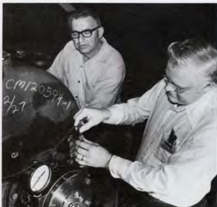
(Above) Charles (Doc) Grimes, 31-year employee, and Leonard Avery, 27-year employee, prepare a LUFKIN gear for testing. The new expansion features one of the finest gear test facilities in the industry. (Upper right) Machine operator Gordon Thomas, 20-year employee, operates a vertical machining center with tool changer in the new gear manufacturing complex. The center was purchased to drill and tap housing components for industrial and marine gears. (Lower right) A LUFKIN marine gear operates in a Seattle State Ferry in Seattle, Washington.
