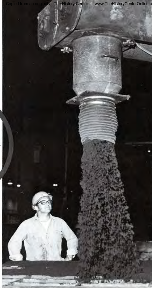
(Left) The no-bake machine in the main bay of the foundry blends sand, resin and catalyst together, and then pours it into the molds. Ferguson developed a new type of mixer head for this mixing process. (Above) Ferguson lined the mixer blades with a plastic-like substance called Tivar 88. The surface reduces the effect of abrasive action.
