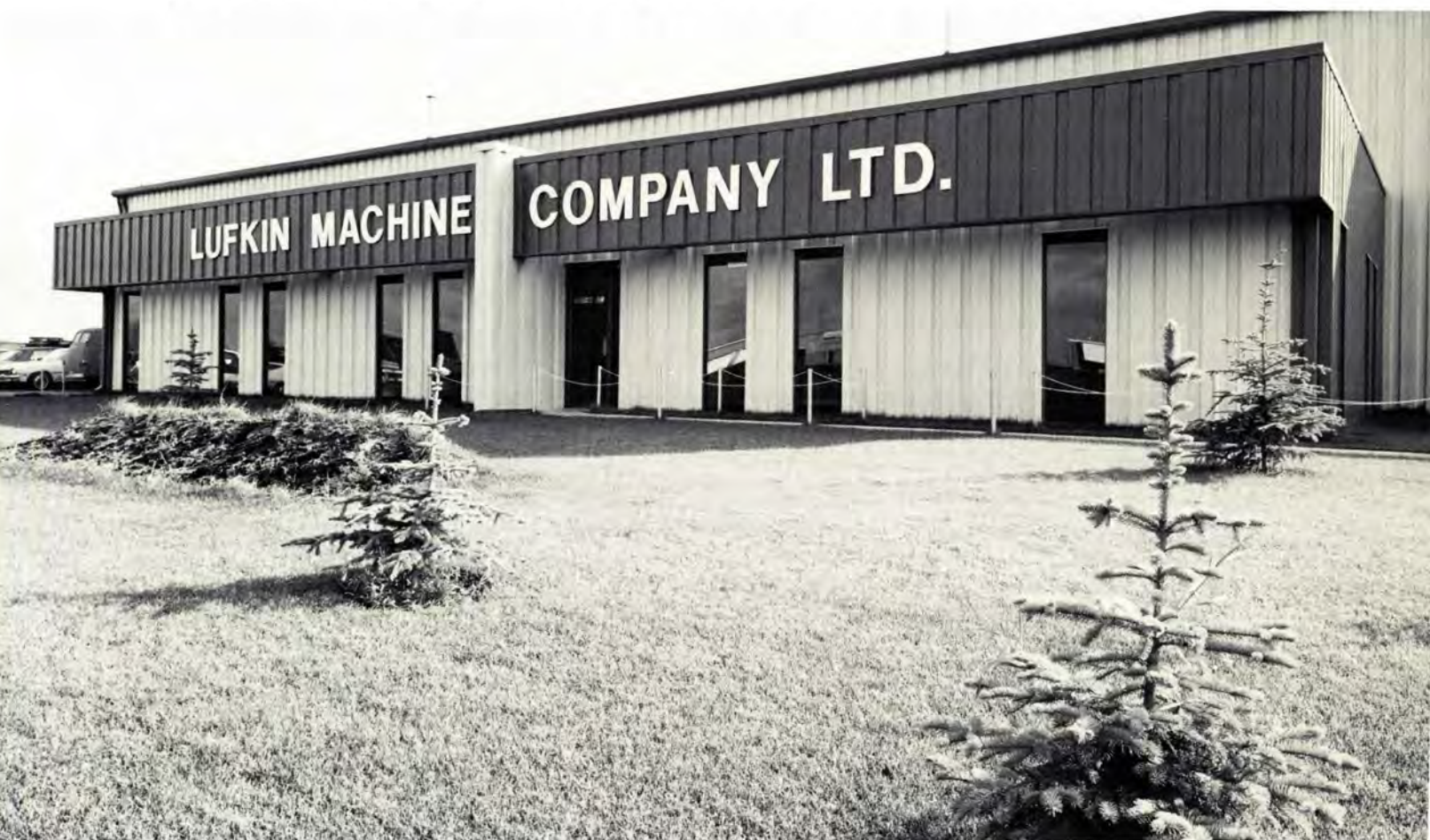
The plant is located 20 miles south of Edmonton, Alberta, Canada in the Nisku Industrial Park. LUFKIN is the park's largest industry.
