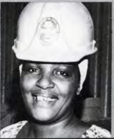
ELLA BANKS Foundry—Core Room 3 years
