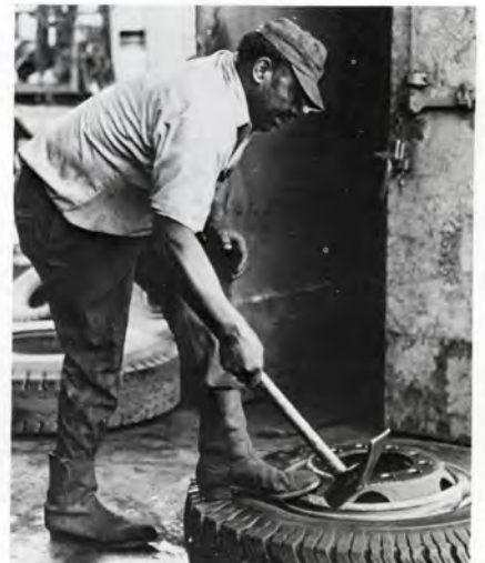
Willie Jones knocks the lock ring off a tire in for repair. If he does not correctly lock the ring back into place after fixing the tire, the air pressure can blow the ring off causing serious injury.
