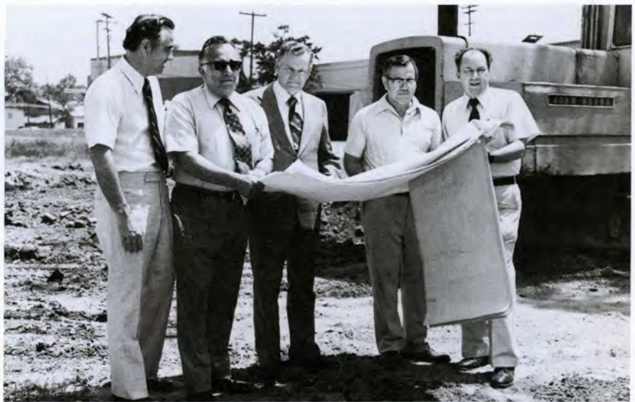
(l-r) Bill Trout, R. E. (Mutt) Barr, R. L. Poland, Stanley Beck and Frank Stevenson look over construction blueprints during the first day of excavation on the new commercial gear building
