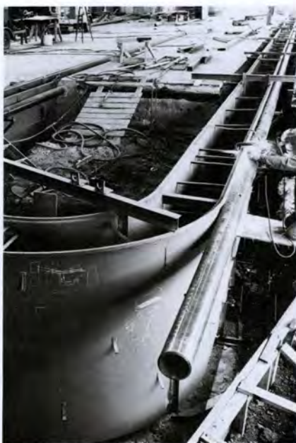
Below-the-floor chip collection and coolant distribution systems complicated foundation work on Old Foundry Renovation project, but will improve efficiency in new building which will house vertical turret lathes and air cylinder-making equipment
