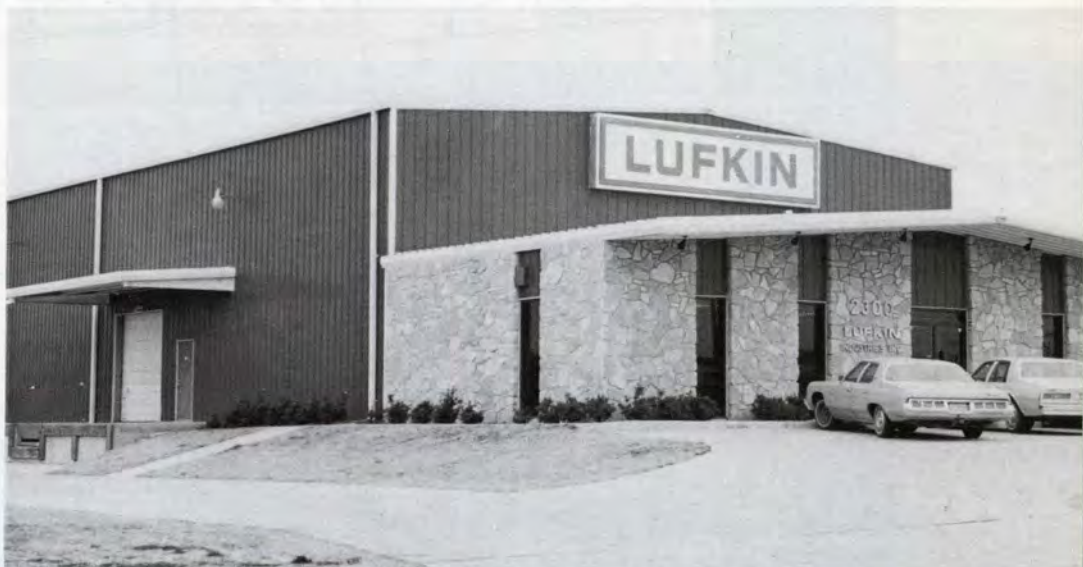
Remodeling, renovating and new construction during 1978 resulted in modernizing trailer branch offices. This is the new Oklahoma City sales and service branch
