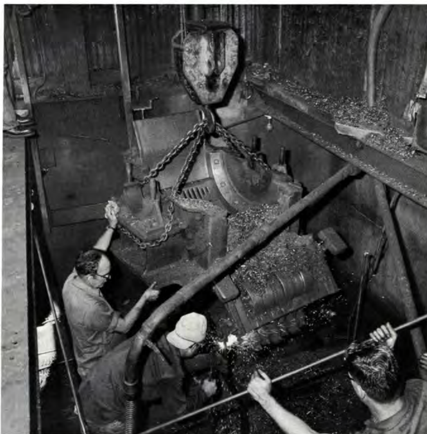
Utility maintenance crews, after two days work, removed the old crusher of the shavings crusher system
