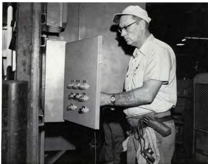
Lee Dunaway, electrical department, wires the master switchboard and in the process of wiring, changes the voltage from 220 to 440
