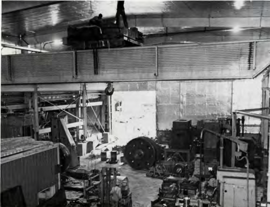
LUFKIN insulated the 8,945 sq. ft. in the north extension of the gear-cutter building
