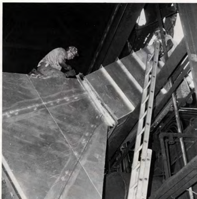
Installing connecting section from outside duct work to shakeout hood (partially seen at left) is Arthur, utility maintenance, and Jimmy Ramey, material control. Jimmy assists with hydraulic crane
