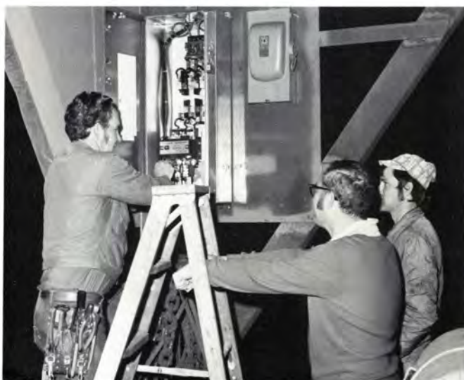
L-r: Estill Holiday, Bill Cantrell, industrial engineering, and Tom Mote install a dust collector, 40 hp, at main bay cupola
