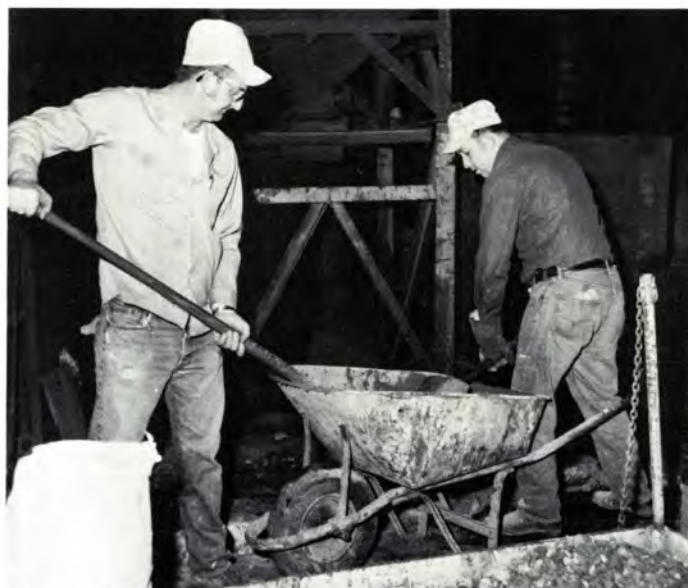
L-r: Alford Hambrick and Terry Allen mix cement for the hopper in foundry
