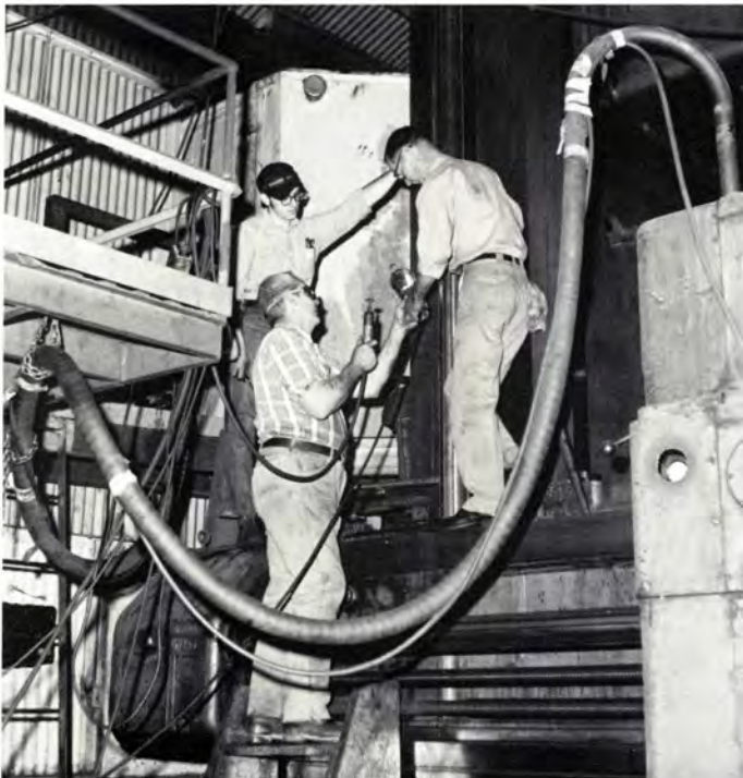
L-r: Gary Luce, Ed Cox, and Norman Arnold replace rail, elevating nuts
