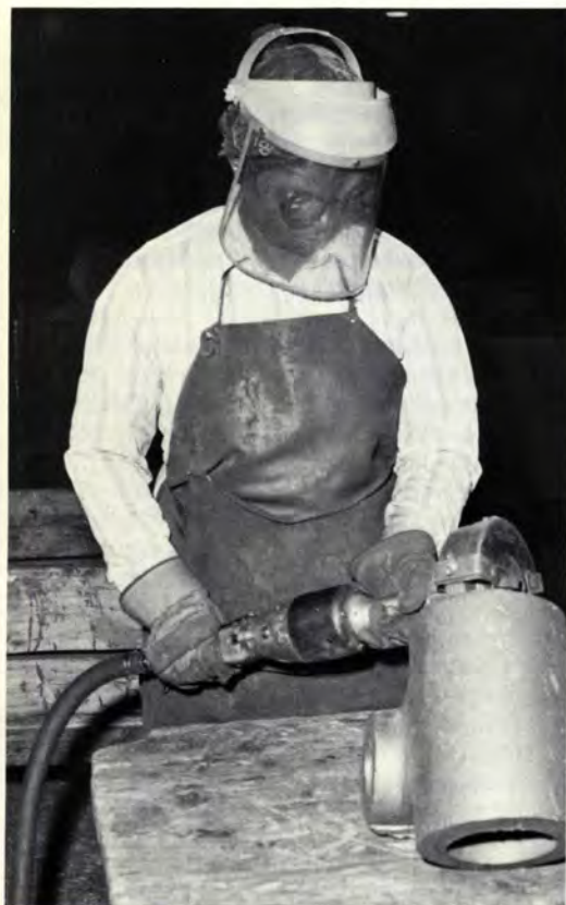
Then castings are sent to Cleaning Room where they are ground by the "chippers and grinders." Ernestine McKelvey (left) uses a floor grinder to clean the "fins" from oil seals and Josephine Patton (right) grinds a bracket. Hand grinders clean hard-to-reach spots on this "box" Lwanda Ligon (center) grinds. All are first shift
