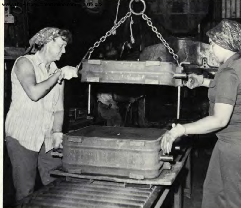
half with a hand crane before closing it and (to right) Evelyn Burney, left, and Mattie Wilson close mold recently packed with green sand. All are molder helpers in the side bay, 1st shift. Next step is pouring molten iron into molds and cooling
