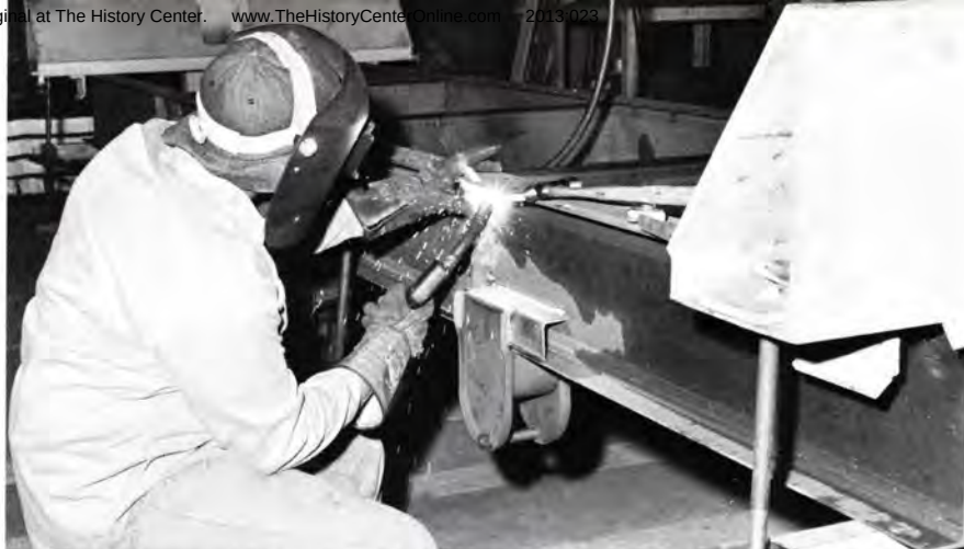
Cloteal Bevil, now also employed in trailer Van Sub-assembly, is welding on the I-beam member of a running gear assembly, used for all types of trailer construction
