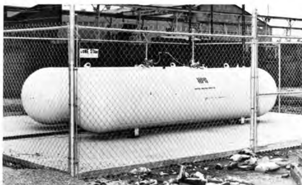
Welding & Structural has switched over to H.P.G. (a liquid, more efficient gas) for all cutting. H.P.G. is one step toward decreasing the demand for natural gas
