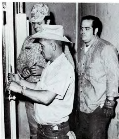
JOHN CLOUDY, front, Nathan McDaniel, left, and John Brittain install cupola control room door for scrubber
