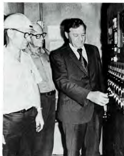
R. L. Poland activates new system. Clayton Jircik, left, and Robert Lang look on
