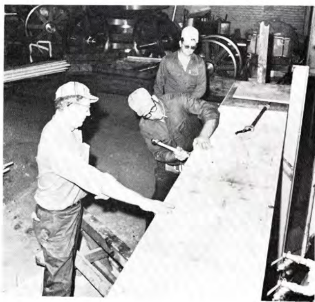
FROM LEFT: William Redd, J. C. "Curly" Modisette and Alford Hambrick nailing forms for Shaft Shop foundation
