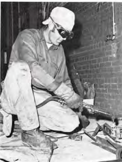
MORRIS MARTIN cuts steel beam, one step in constructing Shaft Shop trench
