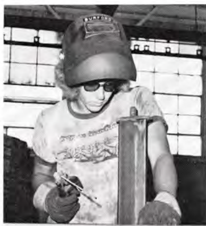
MIKE BURFORD welding tote boxes, for lifting material, in the export area
