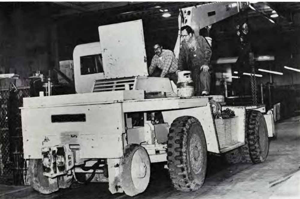
ABOVE: W. C. Green mechanic, right, is servicing a crane, in the plant with Carnuto Rios, a helper on the crew
