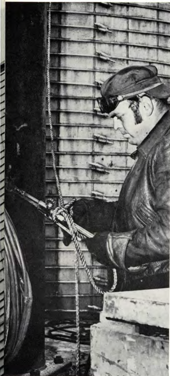
MEANWHILE, on the ground while Steve Edwards is some 45 feet above on the silo, Terry Baird is preparing to send up the burning torch
