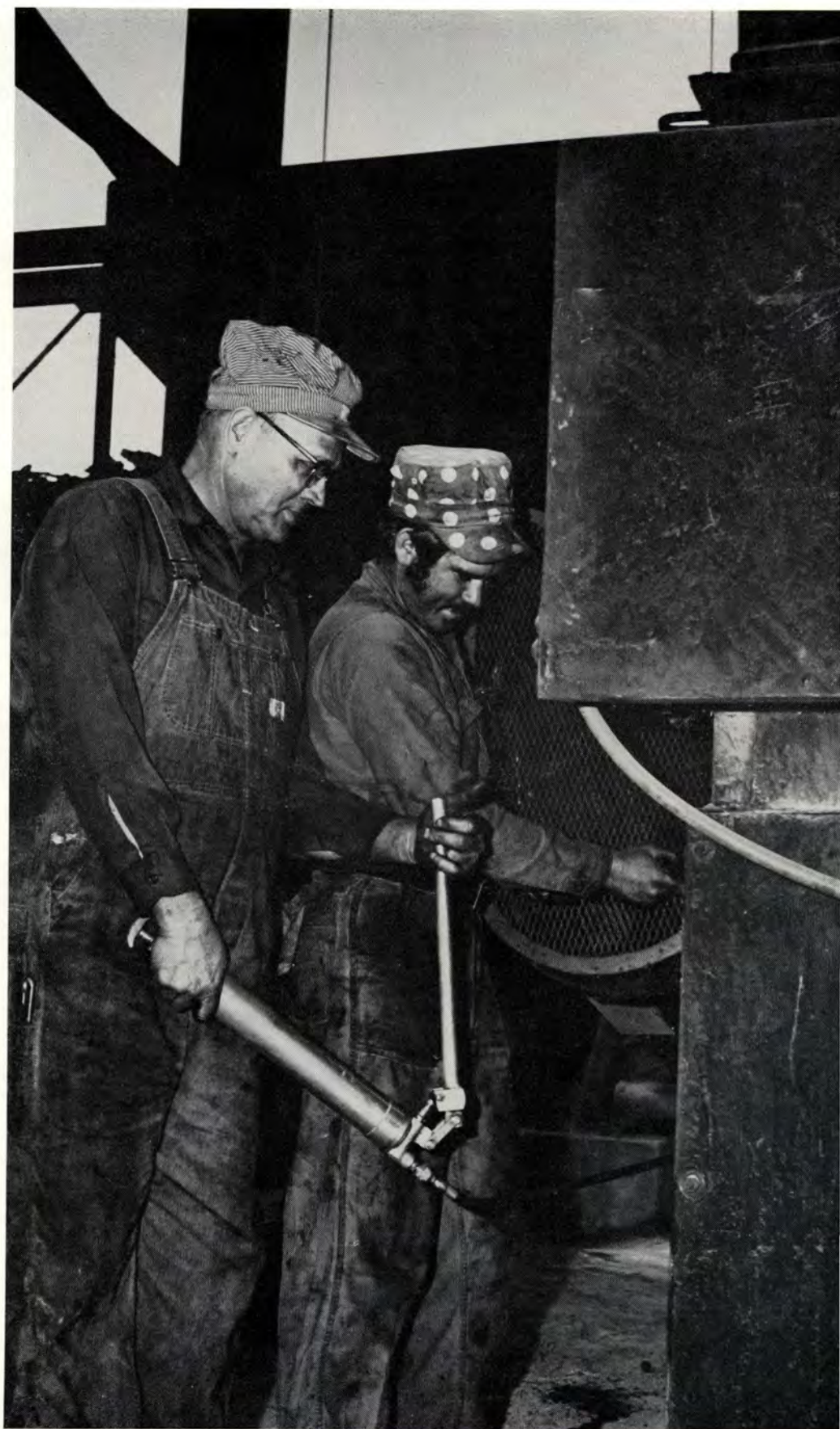
SAM WALL, left, is greasing the lower bearings on the elevator unit of the new sand car unloader as Curtis Hopson lowers a sprocket to tighten the elevator chain
