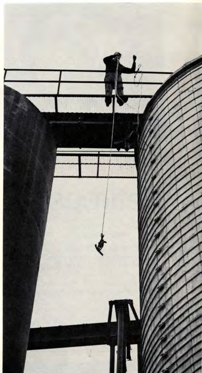
STEVE EDWARDS draws up gear pullers to replace a gear reducer on the foundry's new sand silo belt
