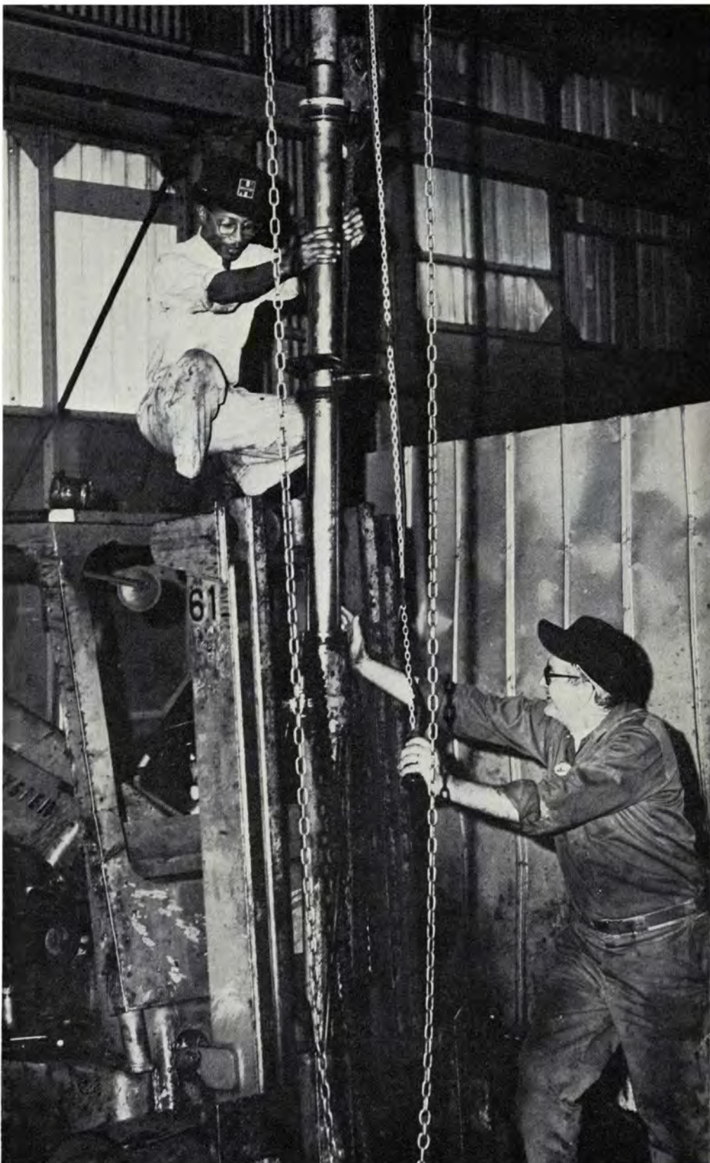
ABOVE: Eddie Mitchell is atop a fork lift truck as he and Robert McNeely overhaul the lift cylinder
