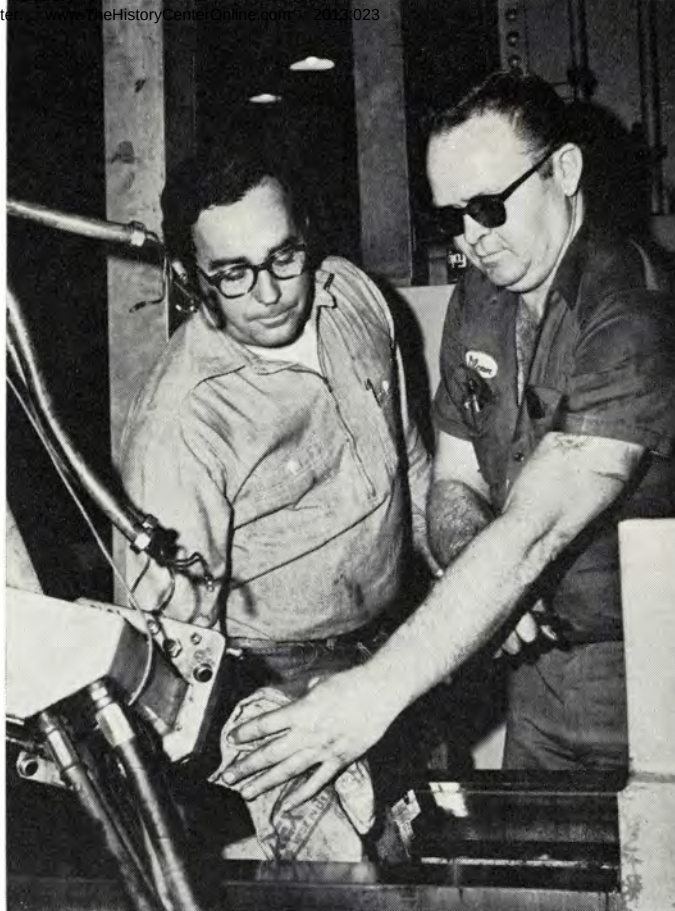
ELTON HENDRY rescrapes and overhauls a milling machine
