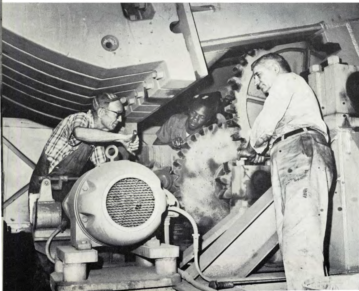
RIGHT: Joe Powell, left, and Glenn Davenport are aligning the Cimx milling machine in the Machine Shop
