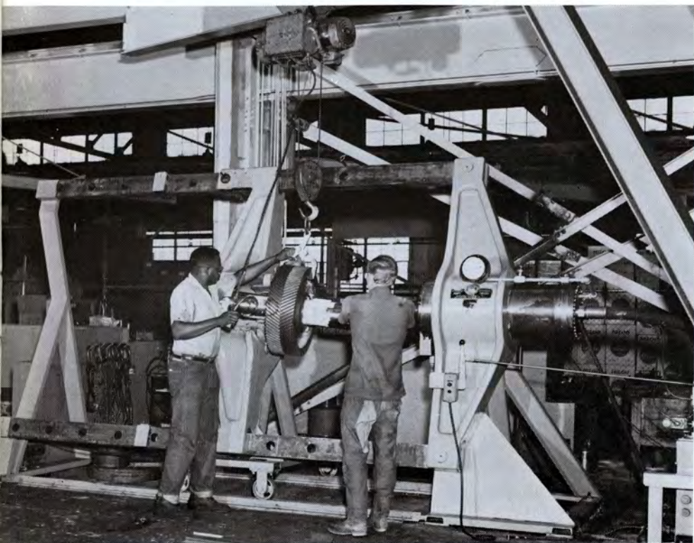
ALSO NEW is this press, where Billy Gardner, left, and Jerry Green are pressing a shaft through a slow speed gear. Later shaft and gear will be set in a box
