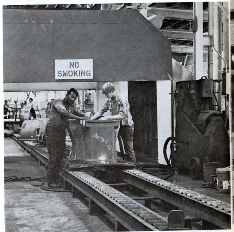
ON THE Assembly Floor a new exhaust system, shown at right has been installed at the gear box cleaning booth. Pictured are W. D. Bryant, left, and Larry Parker. Dust and fumes are drawn from the booth and then expelled through the fan
