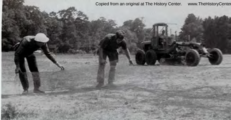
BACKSTOP poles and horizontal stringers were erected as backstop frames. Here Milton Martin, left, and Kent Reynolds unroll chicken wire which was installed at the tops of backstops to catch high foul tips and wild pitches. In background is Tinker Reynolds on Lufkin Industries motor grader levelling an infield area
