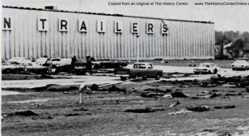
MOST of the roof of the offices was lifted off and dumped on parked cars by the devastating tornadic forces.
