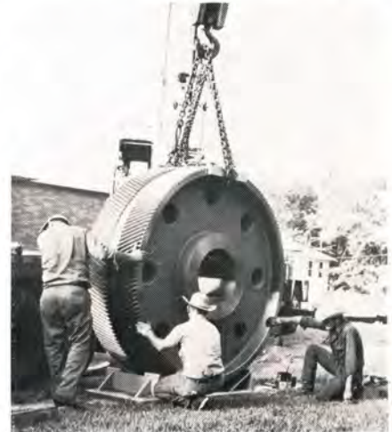
MEMBERS of the Construction and Maintenance crew erected the gear sets. Here they begin the process as A. A. May adjusts the chain. Ervin (Tinker) Reynolds operated the crane.
