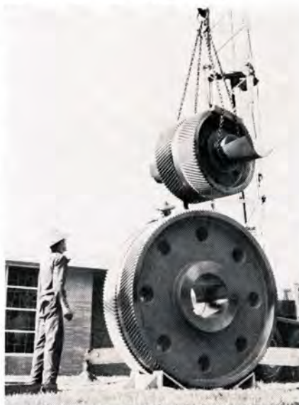
BELOW: THE CRANE lowers the pinion and performs the balancing act. May directs the operation. That's Grimes peering over the top of the gear and he did get his head out of the way!
