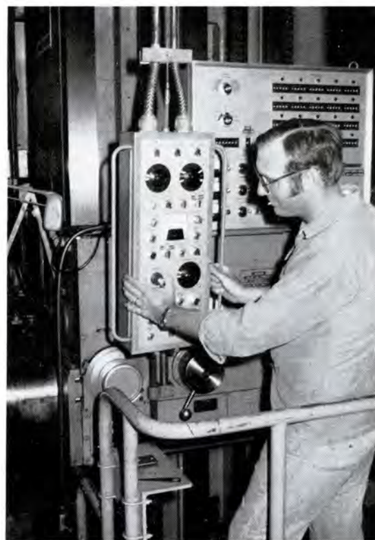
TAPE is being loaded in the "reader" of the control console by Charles Minshew, second shift operator.
