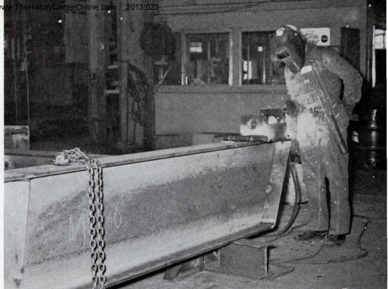
17. P. P. STRINGER, Welding and Structural Shop, first shift, welds the equilizer connection onto the walking beam.
