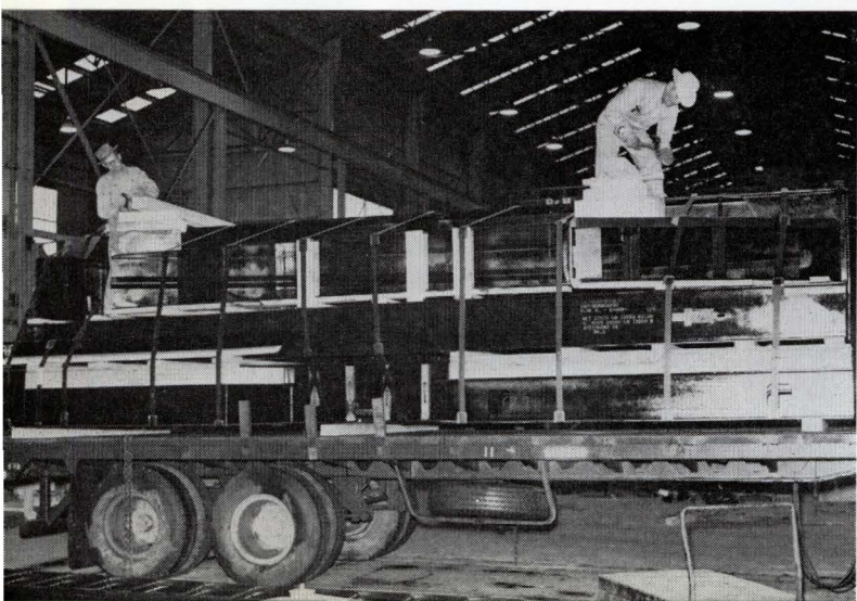
16. HERE a samson post is mounted on a combination positioner and fixture which revolves allowing the welder always to weld in a downward position. Made by Lufkin, this universal welding fixture will accommodate the smallest to the largest post.
