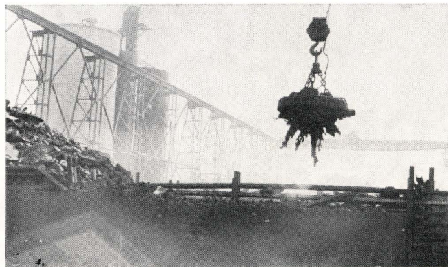
4. METAL for the keels first must be melted in the cupola, a huge furnace which is supplied with tons of scrap metal collected from the yard by this electro-magnet.
