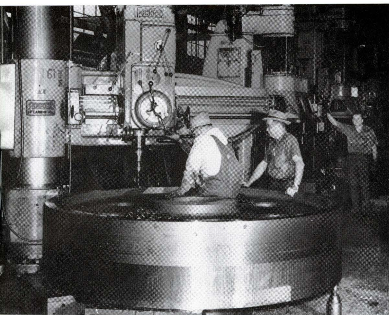
V. A. LUCE is drilling the rim and gear for doweling the rim to the gear. Observing this operation is BOB BUTLER, foreman. Employee at nearby machine is RED McCARTY
