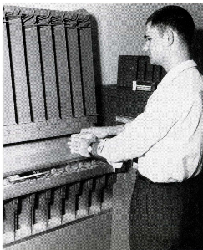
ELVIN LEWIS operates the Card Sorter, a machine capable of sorting 1000 cards per minute
