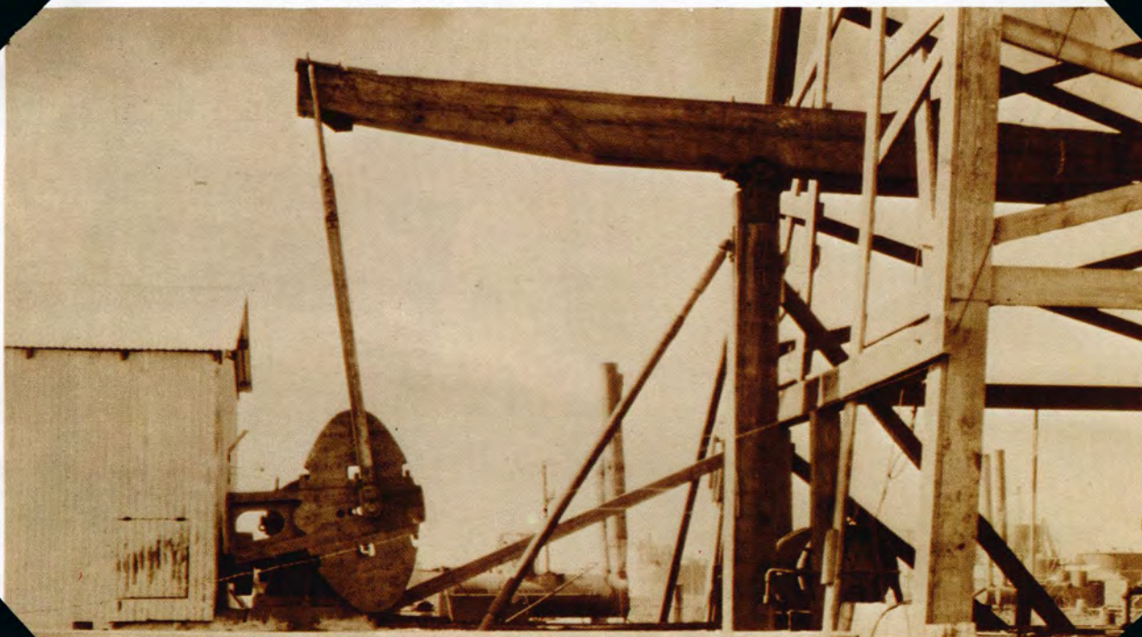
An early LUFKIN pumping unit at Spindletop, Texas, with the Trout counterweight, wooden walking beam, and sampson post.
