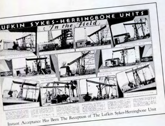
LUFKIN installations as they appeared in the March-April 1930 issue of the Lufkin Line.
