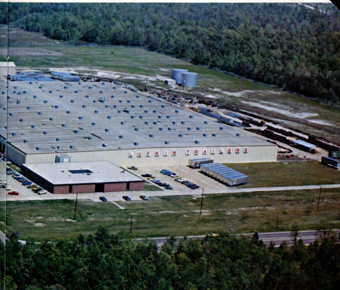
LUFKIN's ultra-modern trailer manufacturing facility with eight acres of production area under one roof.
