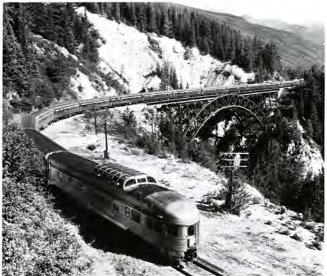
PASSENGERS thrill to crossing of Stoney Creek bridge
