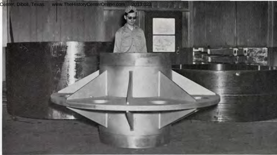
3. THIS photograph shows the center sub-assembly composed of the hub and web plate
