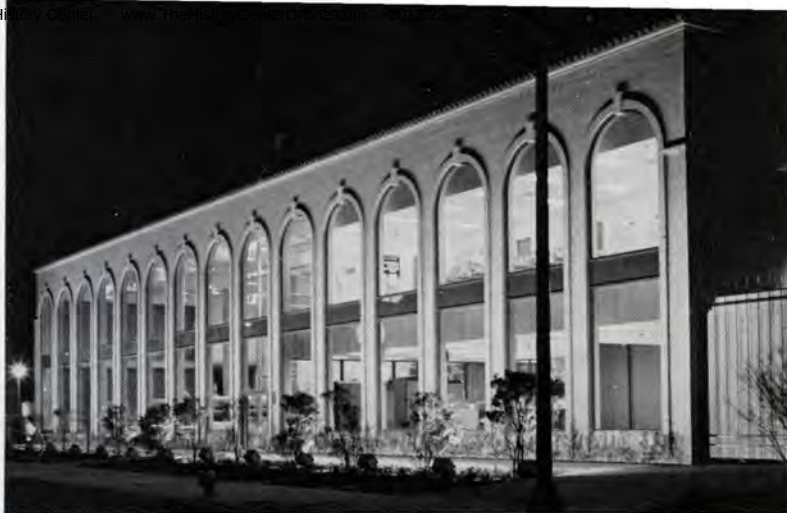
IN KEEPING with Spanish-influenced architecture so abundant in San Antonio, this central heating and cooling plant building adds more beauty to the city.
