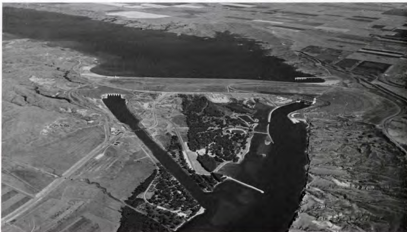
AFFORDING some of the nation's best spiny ray fishing, Oahe Dam is the world's largest earth-fill water barrier. U. S. Army Corps of Engineers Photo
