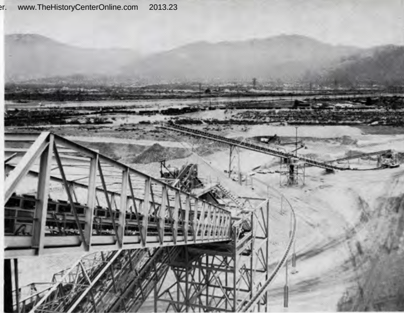
CONROCK'S efficient and smooth running Durbin operation at Irwindale, California utilizes a vast complex of conveyor belts to process daily thousands of tons of rock, sand and gravel. Eight LUFKIN HI-Q Reducers are in service on head pulley conveyor drives, sizes 456DC, 320DA and 160D.
