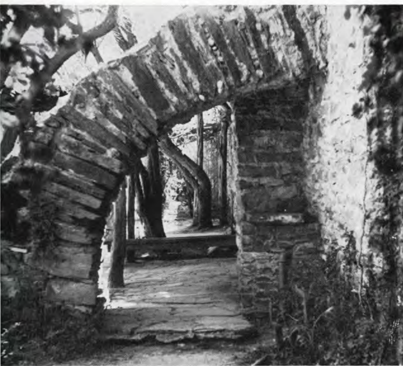
A SERIES of flying buttresses supporting the walls of the granary were added when the church of San Jose with a capacity of almost 1000 persons, was converted to a grain warehouse in 1778.
