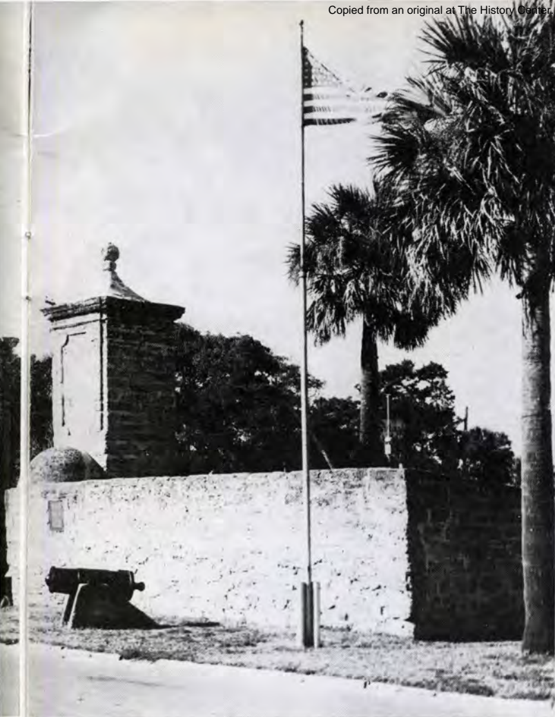
THESE gates were once the main entrance to the city when St. Augustine was surrounded by a coquina wall. During the 400th Anniversary Celebration they will be the passage-way for religious ceremonies, cultural events and festivals
