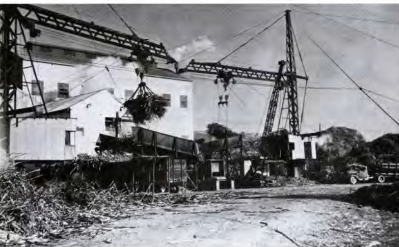
AT the mill, giant cranes feed the cane to grinders where the juice is pressed out, boiled and made into sugar
